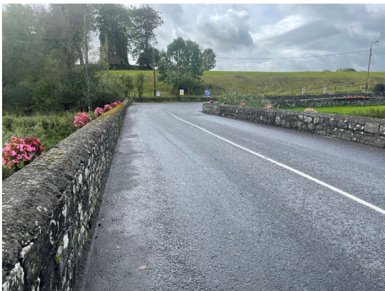
Figure 9 View to South from bridge surface.
