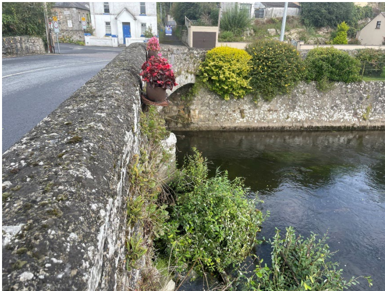
Figure 16 View to North of Splayed Arch AR-07 & CW-06.
