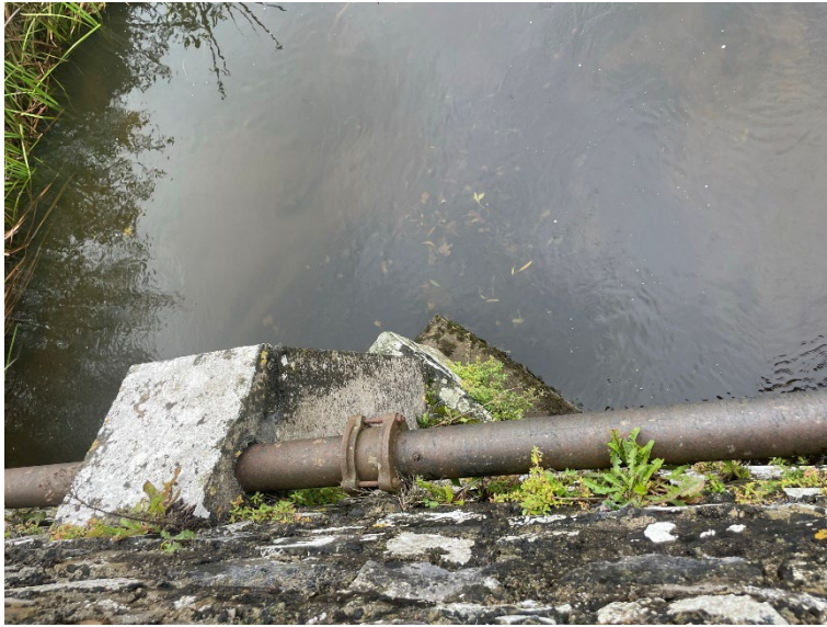
Figure 18 Downstream Cutwater CW-06 with concrete pier supporting existing cast iron watermain.
