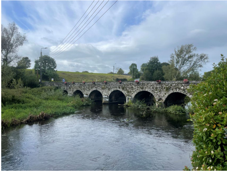
Figure 7 View of Bruree Bridge Upstream Elevation (East)
