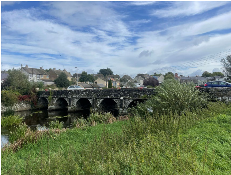
Figure 8 View of Bruree Bridge Downstream Elevation (West)
